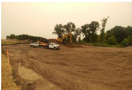
Aug 16/18 Photo facing South East SF 7 Oak Creek crossing (921+250) Excavator building ramp for bridge crossing
