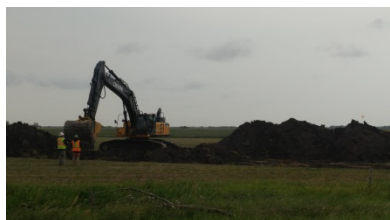
Aug 13/18 Photo facing North Excavator stripping top soil at SF 22
