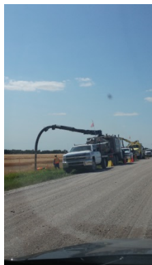
Aug 14/18 Photo taken facing South West Hydro vac crew locating foreign utilities
