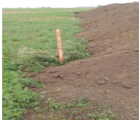
Aug 18/18 Photo facing West SF 22A (KP 942+240) Top soil pile exceeding boundary line.
