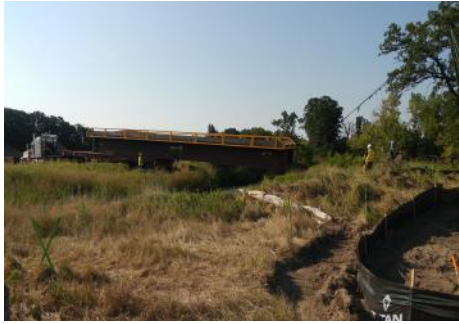
Aug 15/18 Bridge being installed at Oak Creek.
