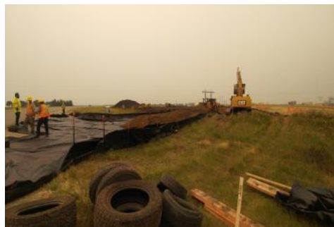
Aug 16/18 SF 21 access Excavator placing soil on to prepped approach
