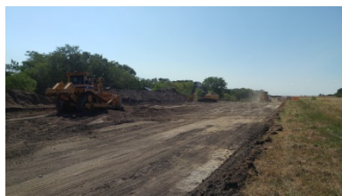
Aug 14/18 Excavator and dozers top soil stripping the east side of Oak Creek crossing
