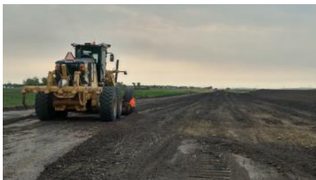
Aug 18/18 Photo facing East SF 22A (KP 942+240) Grader grading the ROW
