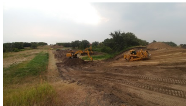
Aug 13/18 Photo facing East Construction crew top soil stripping at Oak creek crossing
