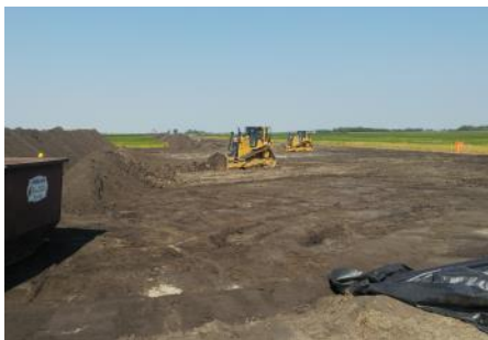
Aug 15/18 Dozers soil stripping ROW.
