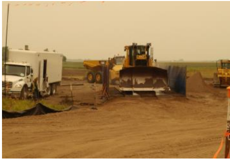
Aug 16/18 Wash station at SF 22 Dozer being fine cleaned and bleached
