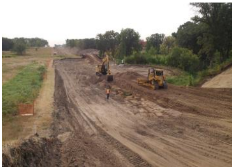
Aug 17/18 Photo facing South East SF 7 Oak Creek crossing (921+250) Excavator and dozer building ramp for bridge crossing
