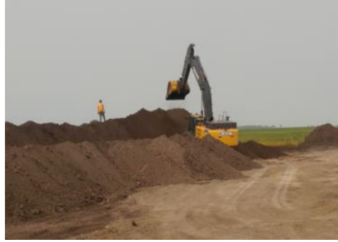
Aug 17/18 SF 19 access Excavator placing moving soil ontop of soil pile
